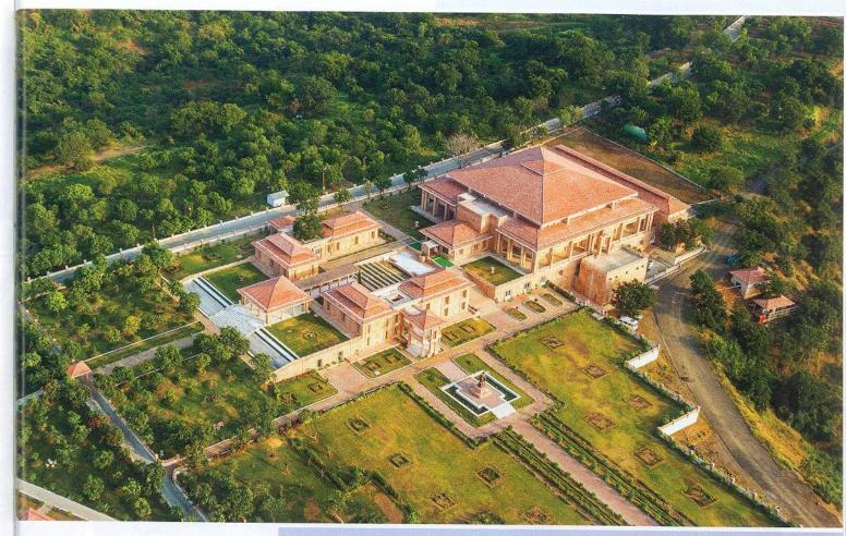
achieving comfortable conditions. Notable features include overhangs and a high-efficiency envelope to reduce solar gains, excellent daylighting and efficient lighting. Energy for the entire complex is derived from onsite renewable sources comprising a solar power plant and a biogas plant. As the project is at a remote location, due consideration has been given to improve the transportation facility for employees, including public transportation access and a car pooling programme.
